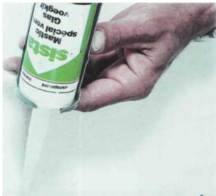
Squeezing the silicone glue onto a sheet of glass. •
